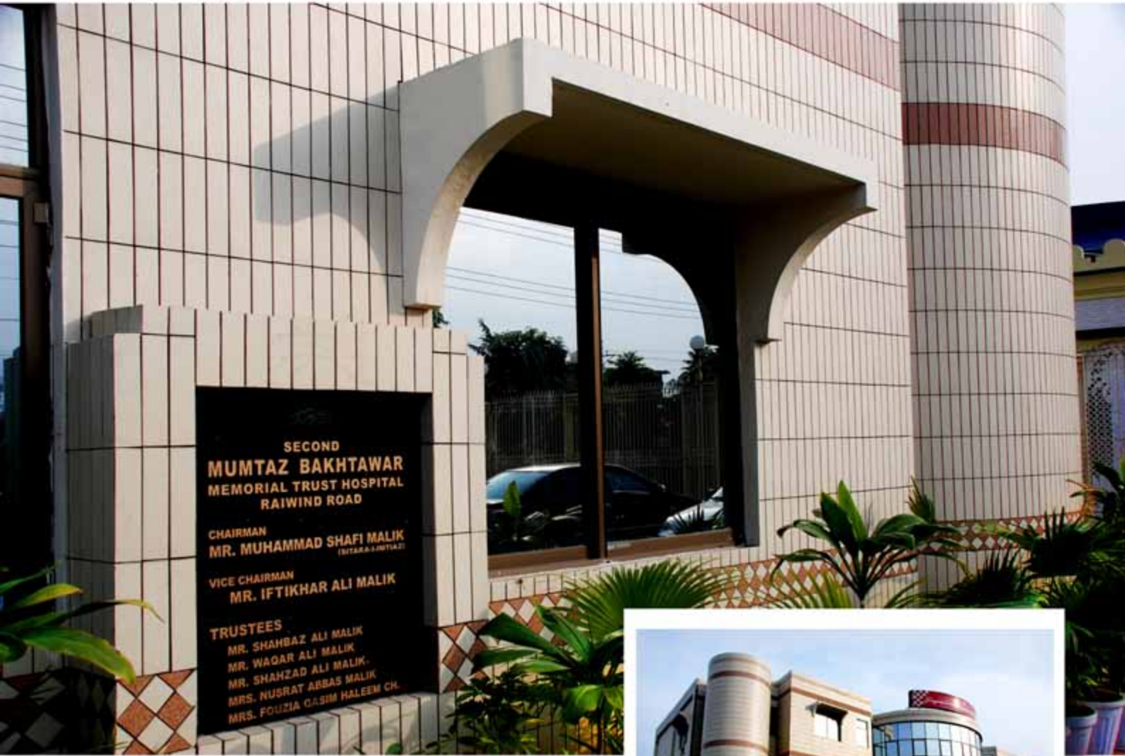
MUMTAZ BAKHTAWAR TRUST HOSPITAL, RAIWIND ROAD
